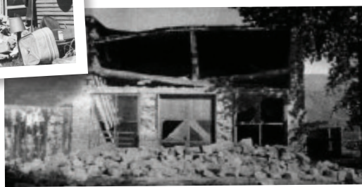
Smaller photos: Damage caused by the M 5.7 Richmond (Cache Valley) earthquake of 1962 (top) and the M 6 Elsinore, Utah, earthquakes of 1921 (bottom). (Photos courtesy of, respectively, Ariel D. Benson, Richmond, Utah, and the F. J. Pack Collection, Special Collections Department, University of Utah Libraries)
