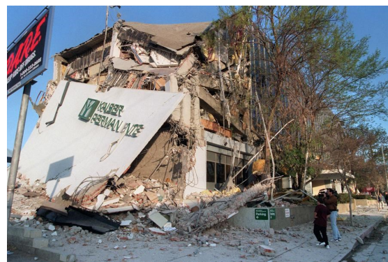
Image: Kaiser Permanente building after Northridge Earthquake Source: Hal Garb, theatlantic.com
