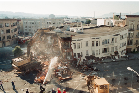
Image: collapsed apartment building in the Marina District of San Francisco following the Loma Prieta earthquake in 1989 Source: AP Photo/George Nikitin
