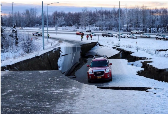
Image: Damage from the Anchorage, Alaska earthquake Source: Donovan Johnson
