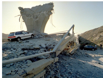
Image: Destruction from the Northridge earthquake Source: LA Times
