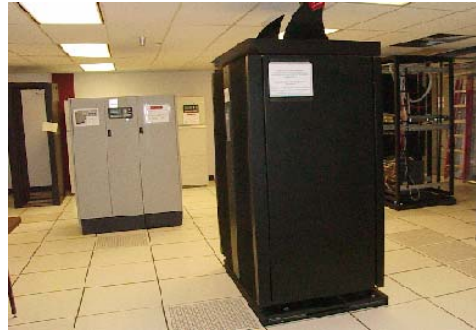
Computer Servers Mounted on ISO-Base Platform
